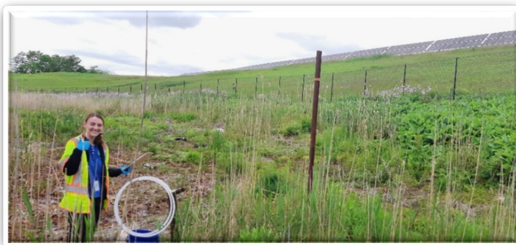
Developing a monitoring well at a landfill
